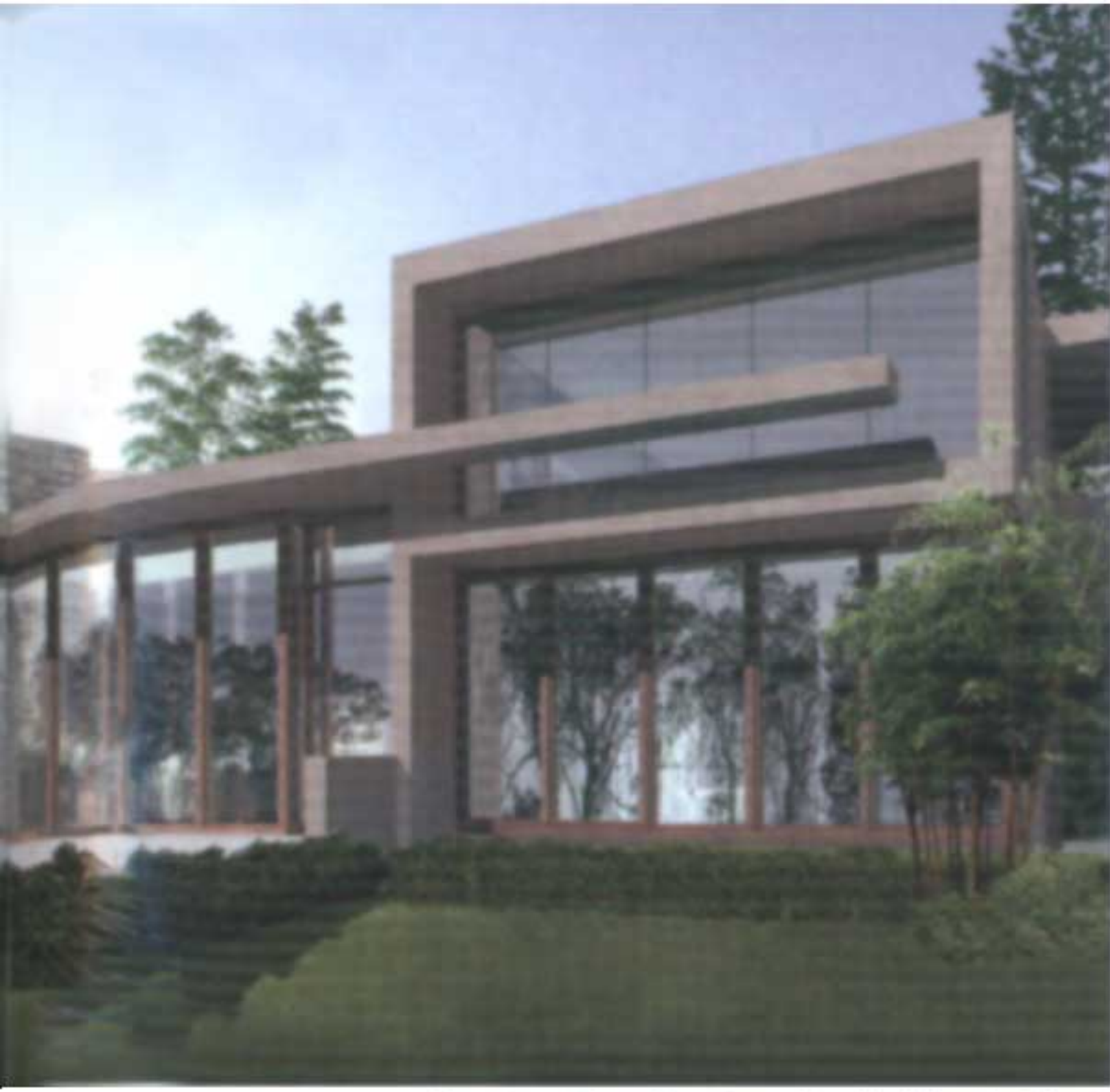
Courtesy Olson Sundberg Kundig Allen Architects
